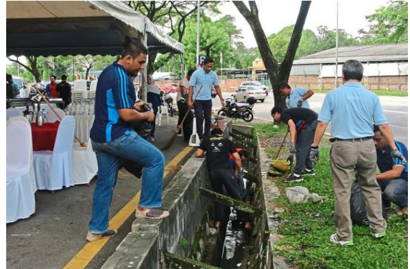
DBKL and Unitab Medic employees unclogging and cleaning the drains.
